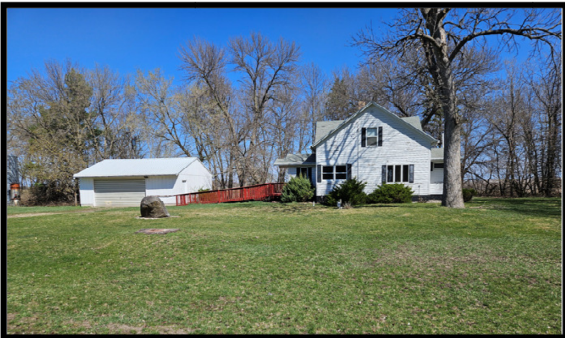
House & Detached Garage
